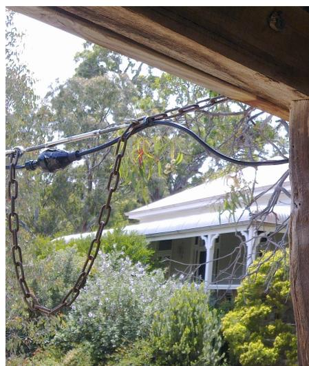
**Lamp holders with globes fitted, MUST NOT be pointing upwards, as this will collect rain and trip out your circuit breakers.**
